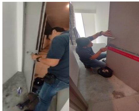
Modification of Staircase Locks
