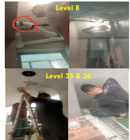
Plumbing Repair Works
